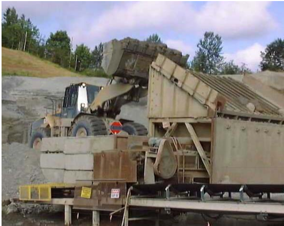
Figure 2: Loader feeding shaker
