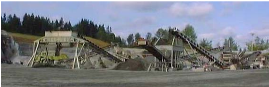
Figure 1: Portable screening and crusher operation
